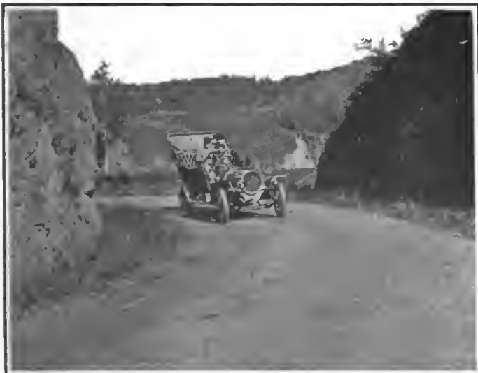
Sharp Turn in the Military Road Up Grade in a Rocky Cut.
